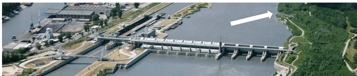
Figure 41: Freudenua Hydropower Plant downstream of Vienna with natural fish ladder on the right side of the picture (picture sources: https://www.verbund.com/de-at/ueber-verbund/besucherzentren/freudenau )
