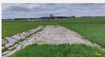
Figure 29: Retention basin with outflow structure in upper picture left side and dam overflow area in below image (Picture source: Sonja Hofbauer)
